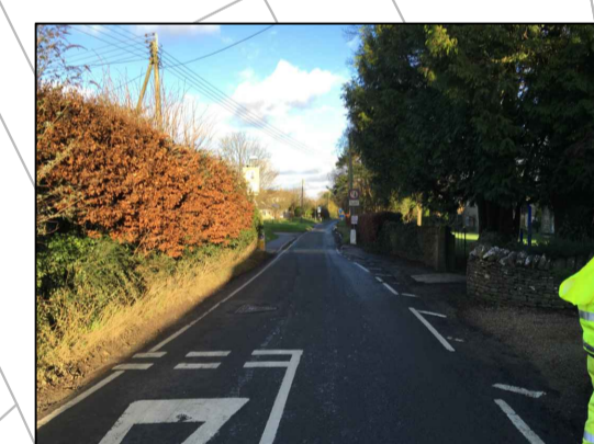
Vegetation clearance to provide suitable visibility of signage
