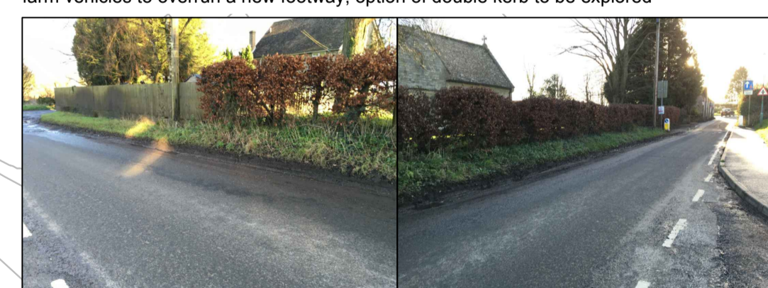
Carriageway too narrow (<5m) to accommodate footway so a land purchase required to accommodate a 1.5m footway. Narrow carriageway could encourage vehicles - particularly farm vehicles to overrun a new footway, option of double kerb to be explored
